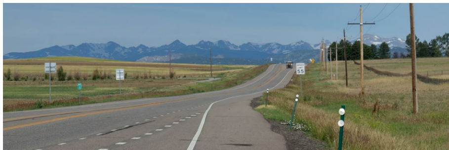
CO 52 (MP 3) looking west along corridor
