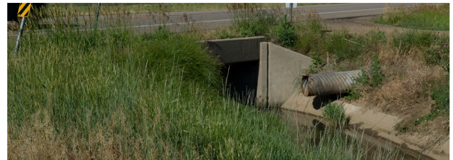
Culvert and drainage pipe at the west end of CO 52
