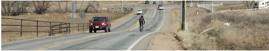
Insufficient shoulder width for multimodal use
