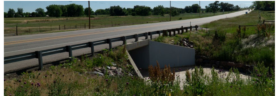
Looking west at box culvert conveyance in Boulder County
